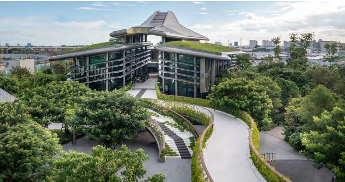
Grand entrance and drop off. Photo credit: Rungkit Charoenwat
