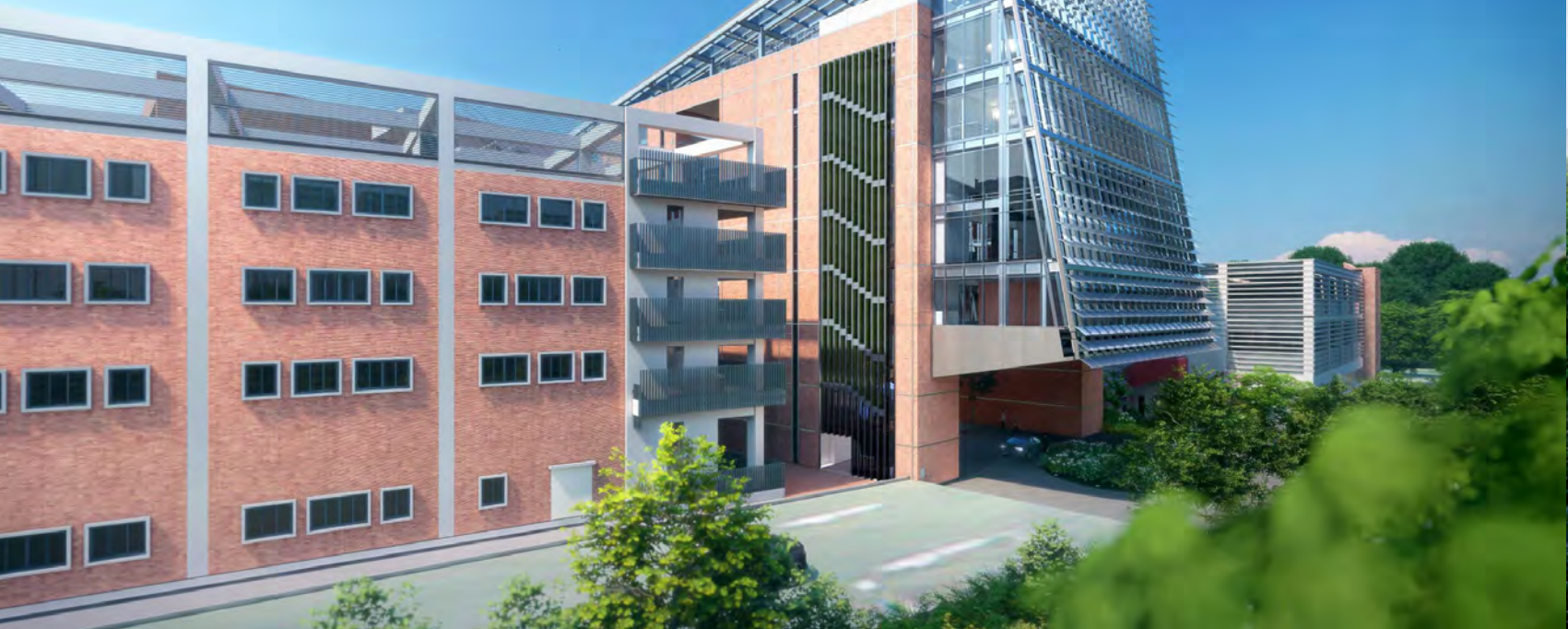
Facade and drop off.
